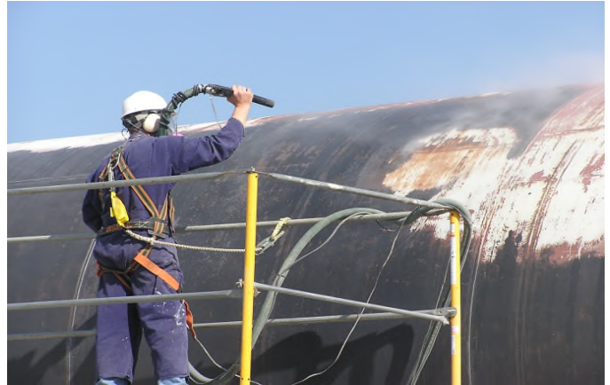
Removal of industrial coating and rust from active propane tank.
