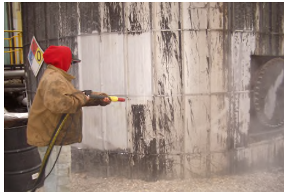
Removal of asphalt from thin gauge tin
